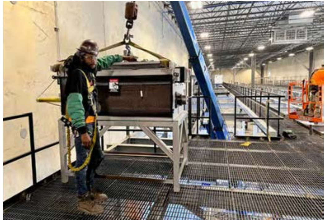
Millwright team rigging 3,000 lb motors for elevated conveyor line at a new UPS regional hub
