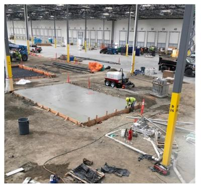
The scope and schedule for the project required a nearly 24-hour a day work cycle: excavation, grading and re-bar by day, and pouring by night.
